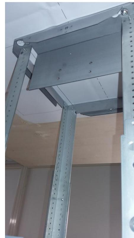
Remove the protective trim from the upper and lower duct to get access to the fixing screws and remove the ducts /
